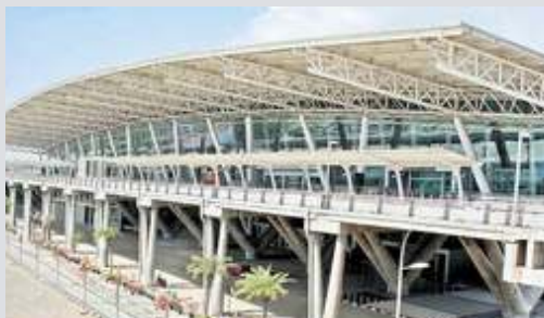
Chennai International Airport
